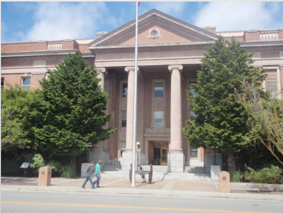
Skagit County court house
